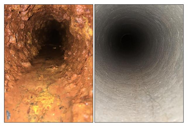
Above left, 4" tuberculated watermain before cleaning. Above right, "best in class" surface preparation by Tomahawk for superior long-term, leak-free liner application.
