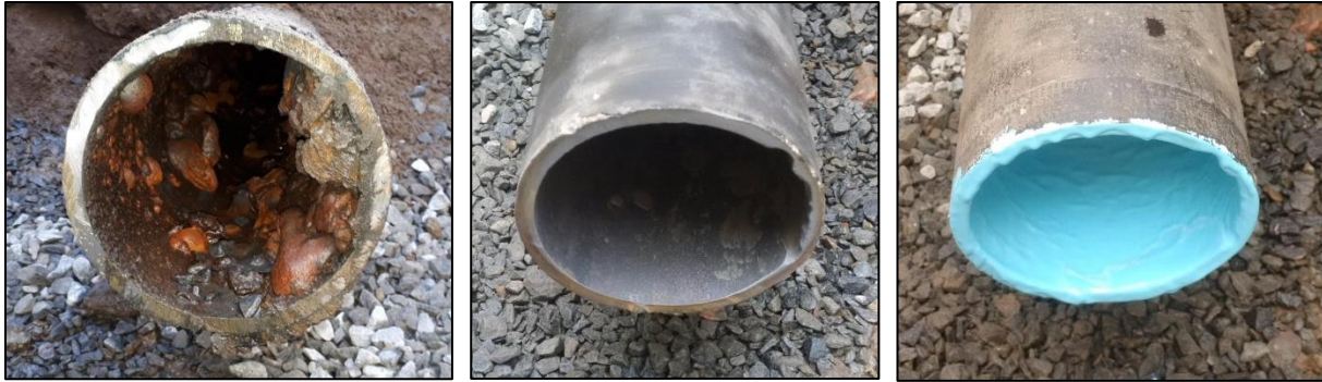
Pictures: Above left, watermain before cleaning, center, after cleaning with Tomahawk, right, after lining with Tomahawk BluKote™.
