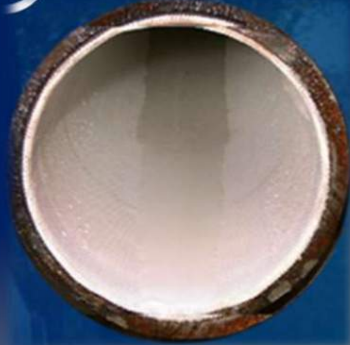
Cured-in-place pipe (CIPP) $400 - $700/meter lining
